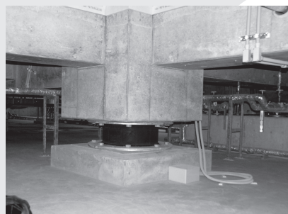
Seismic isolation structure at Aso Medical Center.
